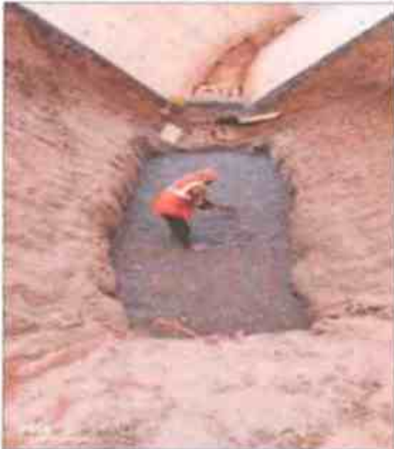
In-line Rainwater Harvesting Pits
