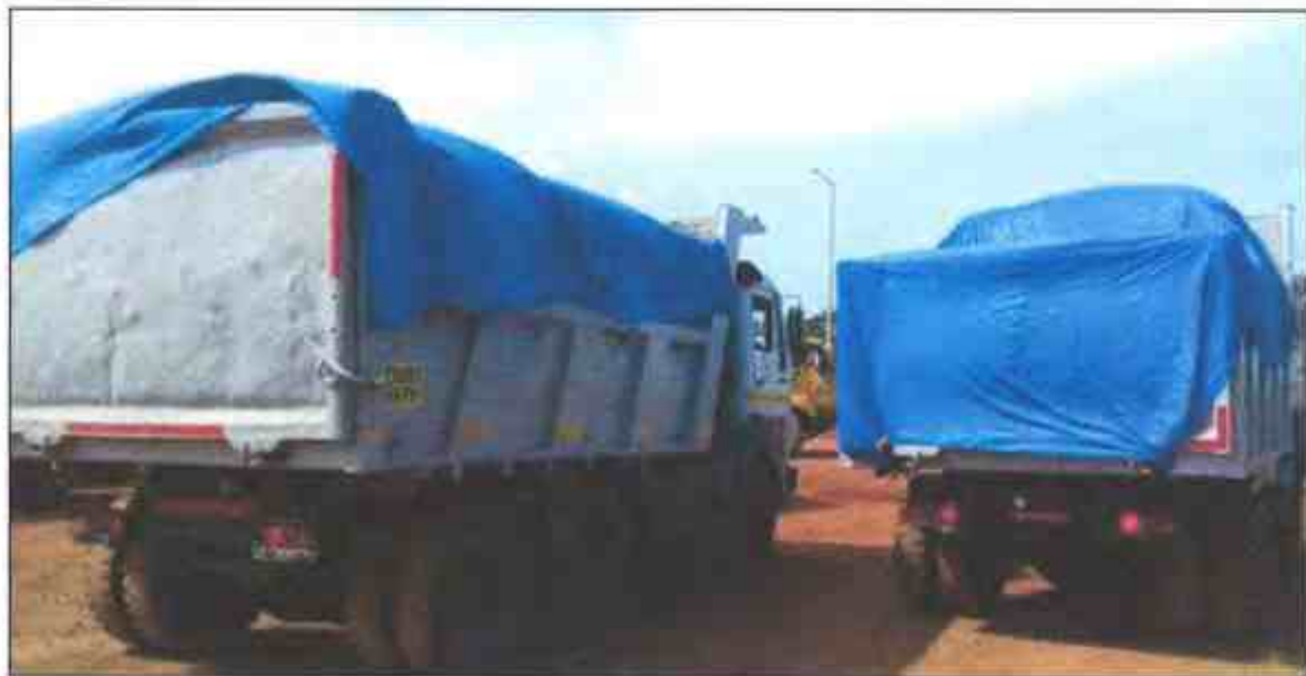
Excavated materials transported by covering with tarpaulin sheet
