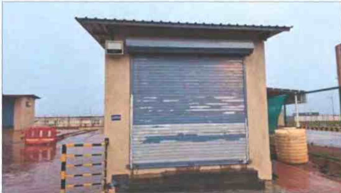
Hazardous Waste Storage Facility
