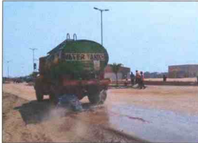
Water Sprinkling on Unpaved Haul Roads
