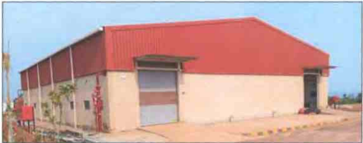
Integrated Solid Waste Management Facility
