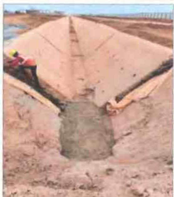
In-line Rainwater Harvesting Pits
