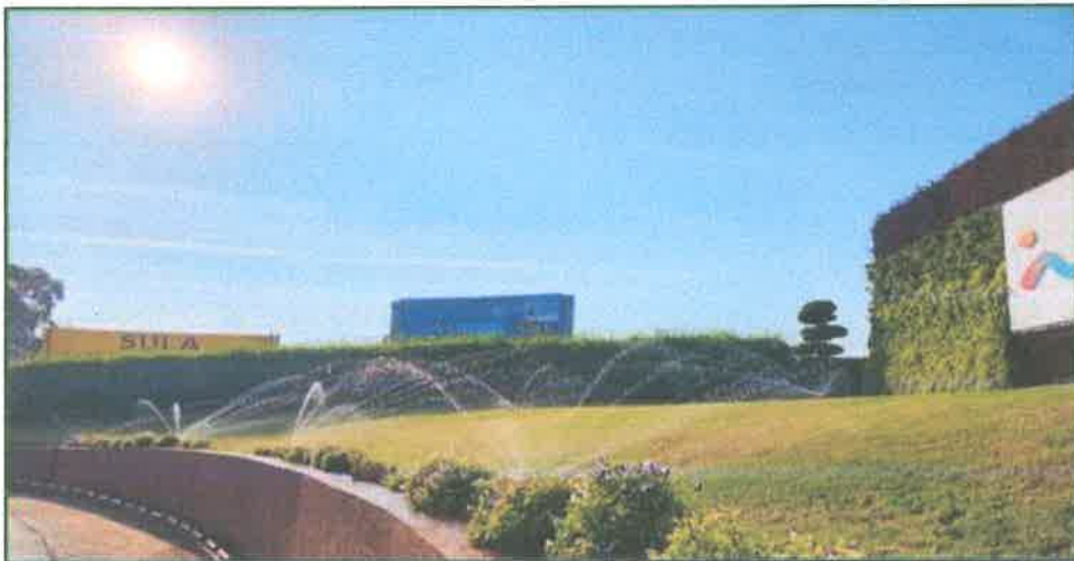
Sprinkler Irrigation for Landscaping & Avenue Plantation
