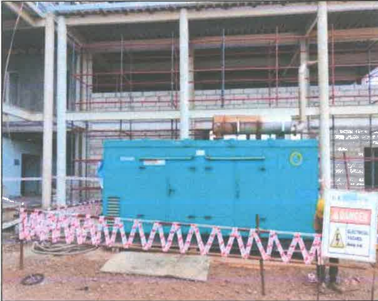
DG Set with adequate Stack Height
