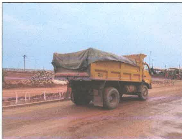
Excavated materials transported by covering with tarpaulin sheet
