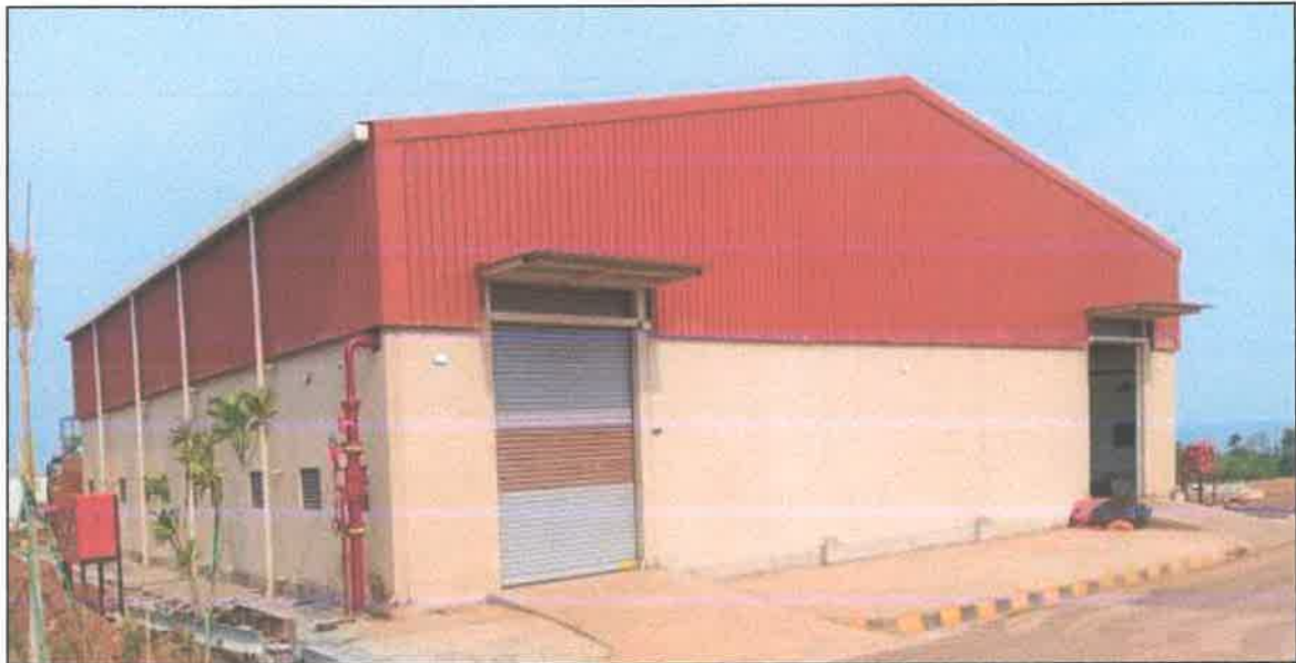
Integrated Solid Waste Management Facility
