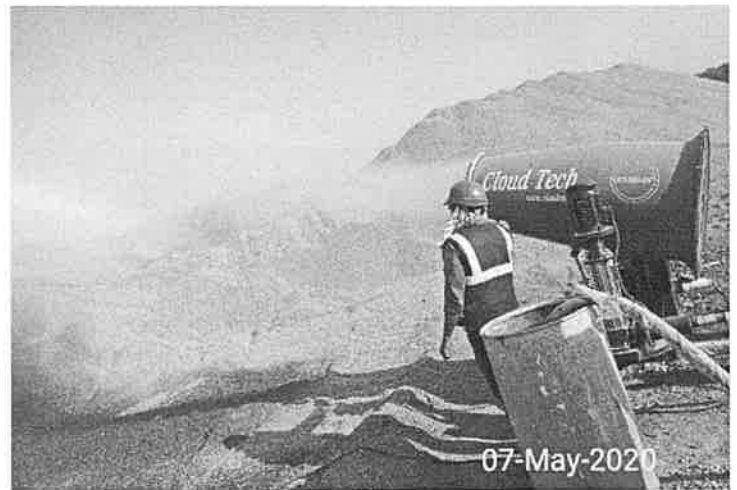
FOG CANNON AT MATERIAL STORAGE AREA OF WMM
