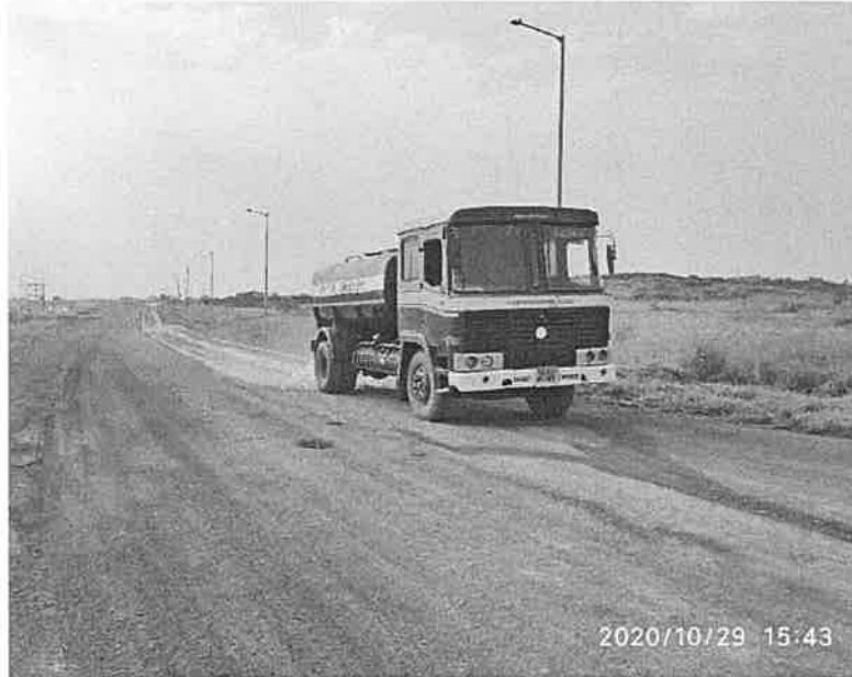
WATER SPRINKLING ON UNPAVED HAUL ROADS
