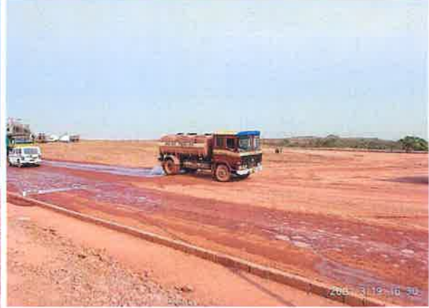
WATER SPRINKLING ON UNPAVED HAUL ROADS
