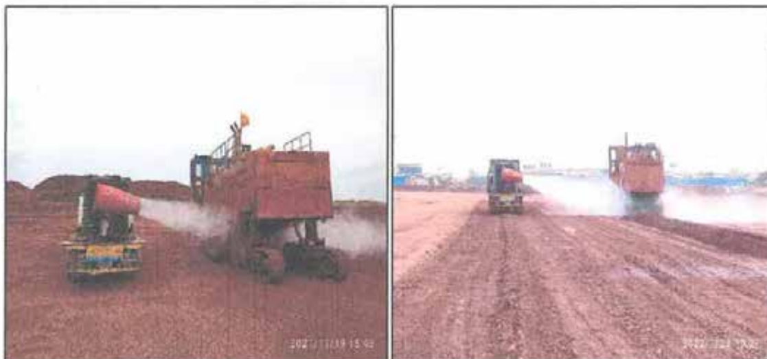
FOG CANNONS DEPLOYED AT EARTH WORK AREAS
