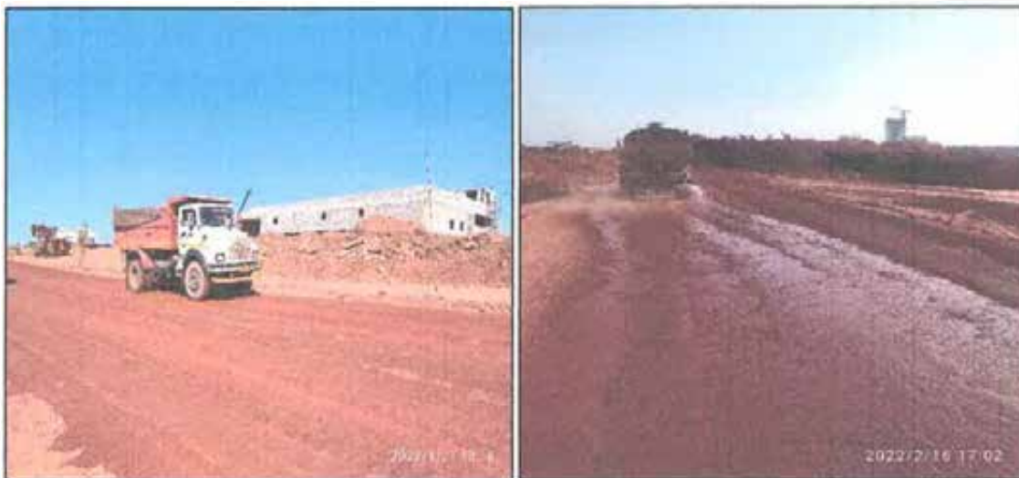
WATER SPRINKLING ON UNPAVED HAUL ROADS
